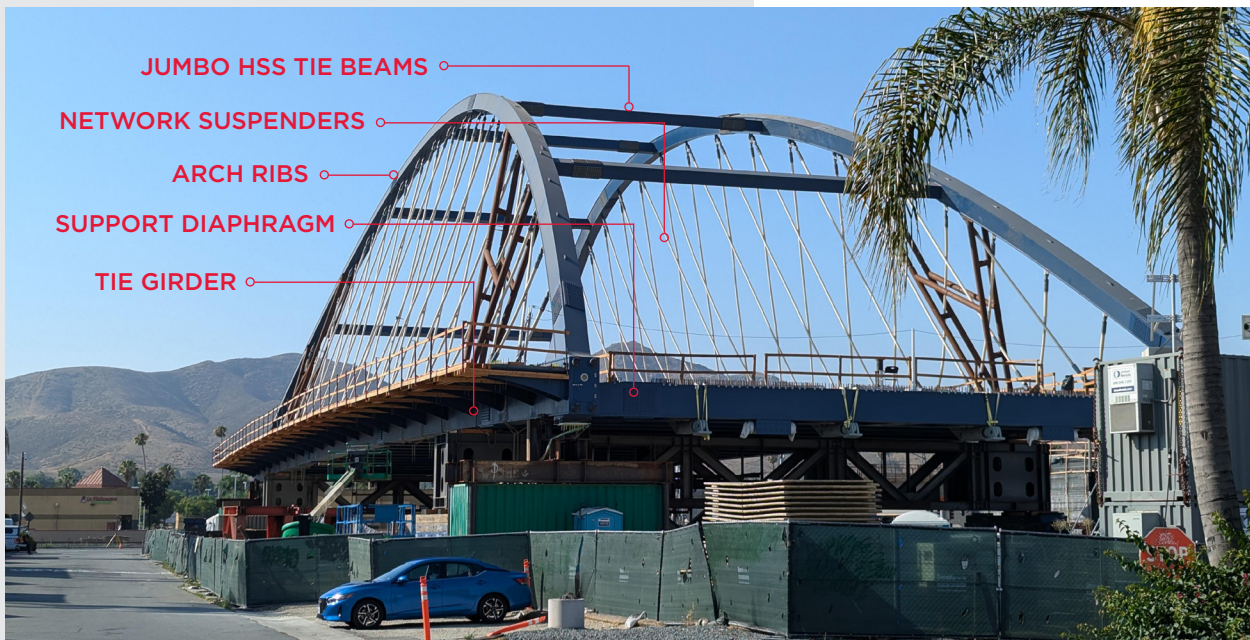
Overall shot showing the various structural elements.
